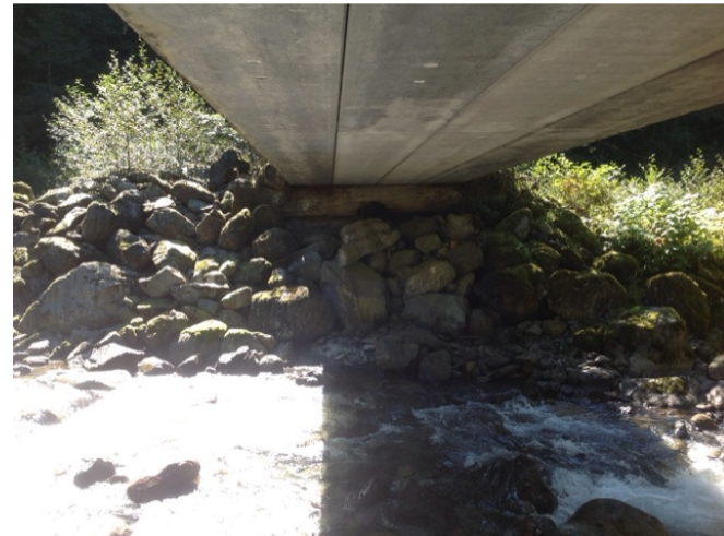
Left Bank Abutment when facing downstream
