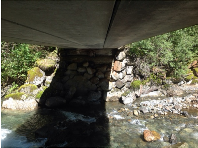
Right Bank Abutment when facing downstream
