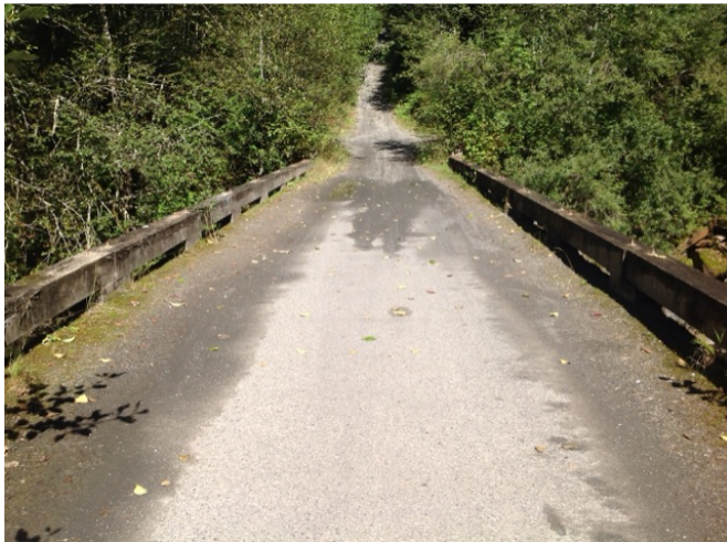
Deck - asphalt cover
